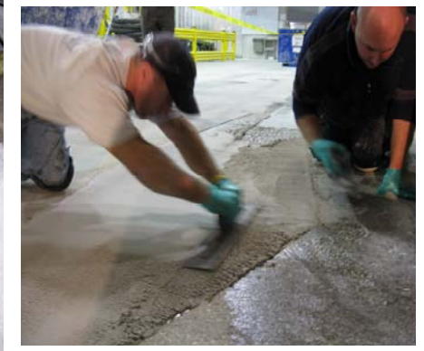
Troweling on the Floor Tech RS.
