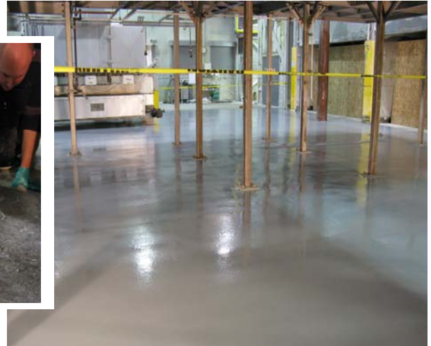
Finished project protected with Floor Tech HB
